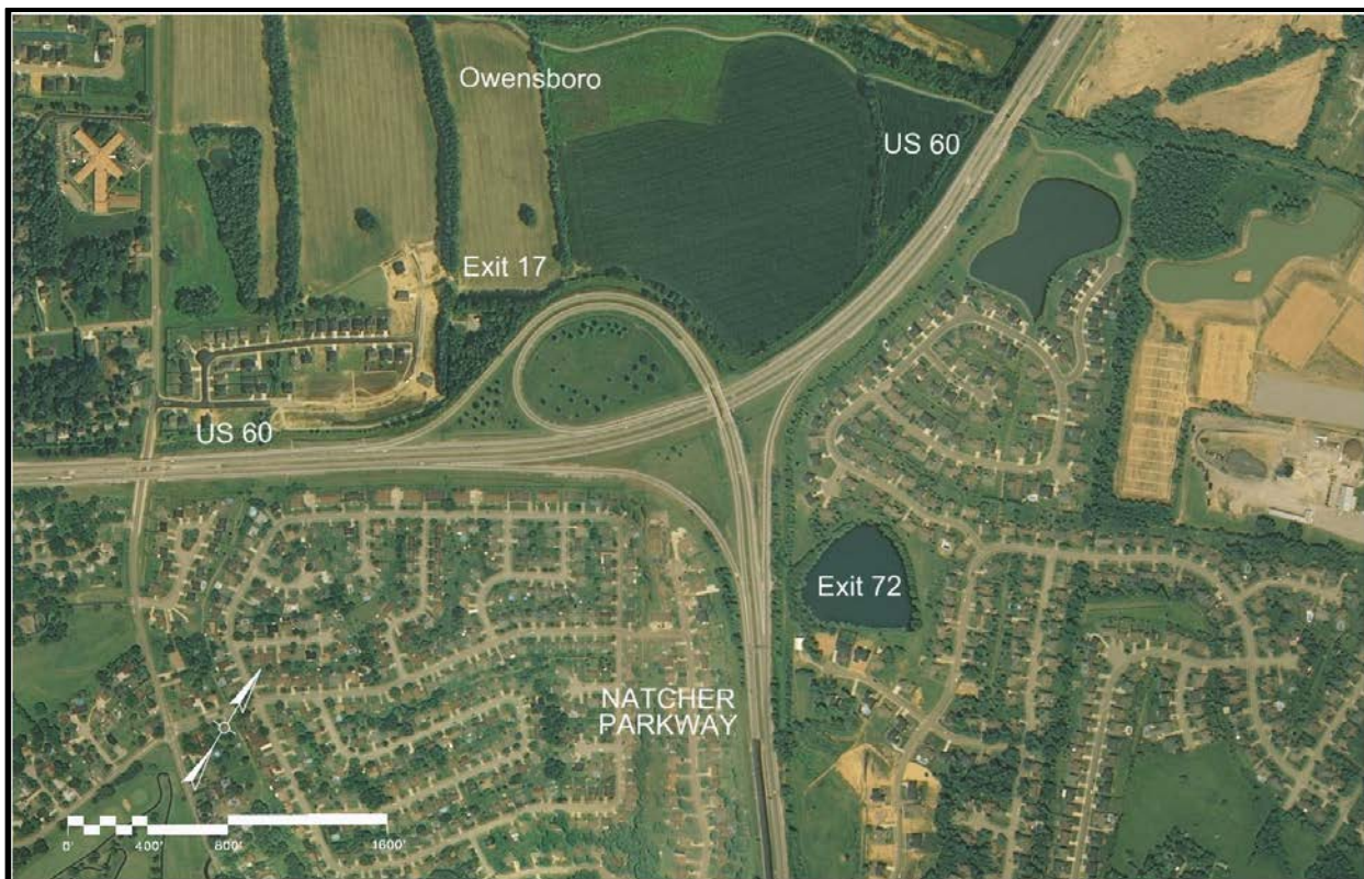
Figure 5 Natcher Parkway / US 60 Trumpet Interchange
